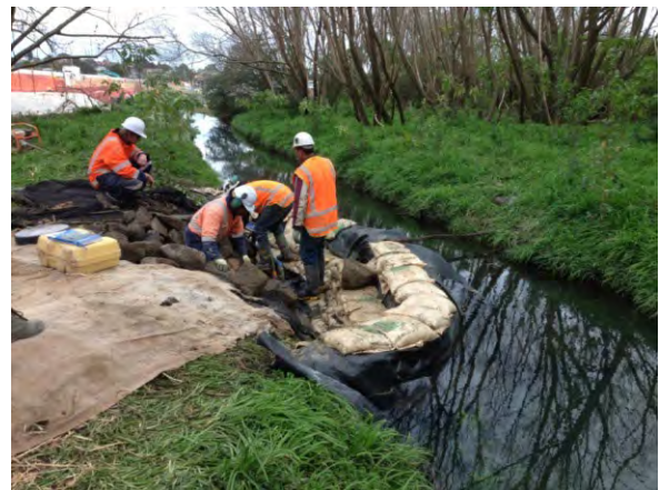
Figure 123: Sandbag coffer dam installed to complete stormwater outfall
