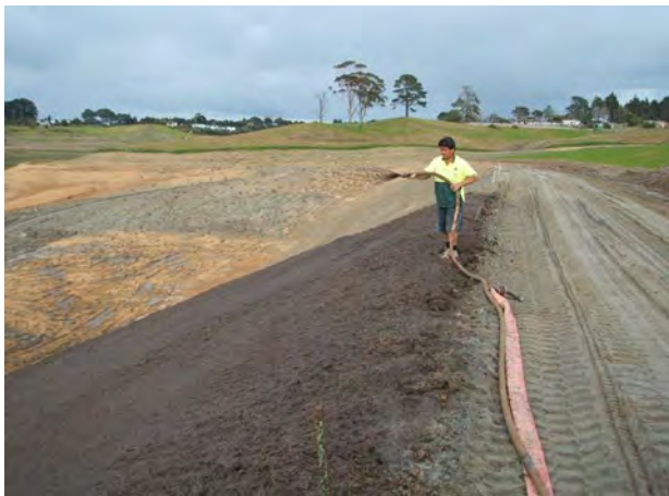
Figure 55: Hydromulch application
