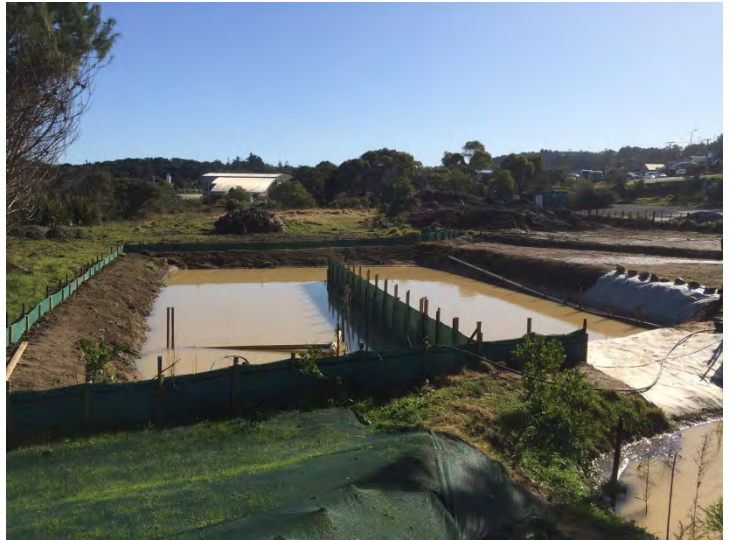
Figure 68: Example of baffles
