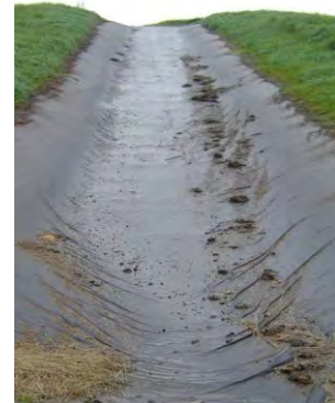
Figure 31: Geotextile lined flume
