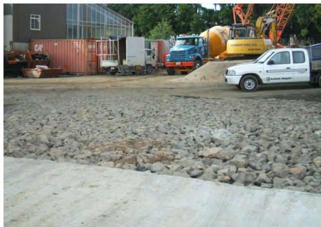
Figure 35: Stabilised entranceway
