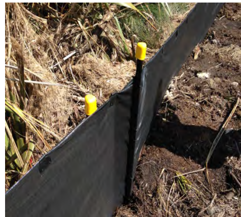
Figure 81: Silt fence joins. Left hand photo shows battens used to join the lengths. Right hand photo shows doubling over of fabric at end around the waratah
