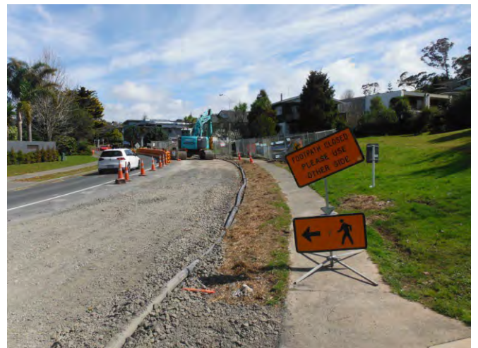
Figure 110: Use of stabilisation products and progressive stabilisation
