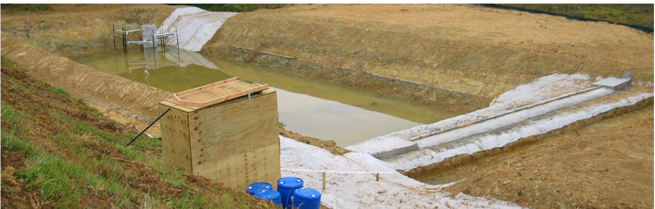
Figure 10: A typical earthworks construction site
