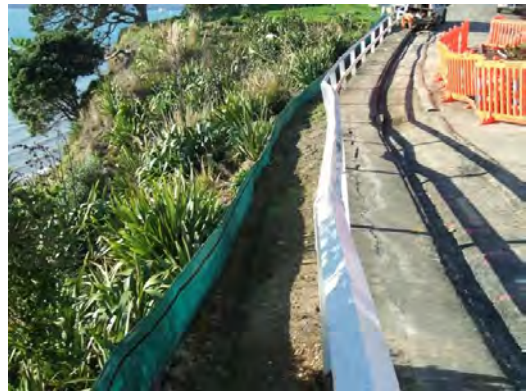
Figure 80: Silt fence installed on edge of works
