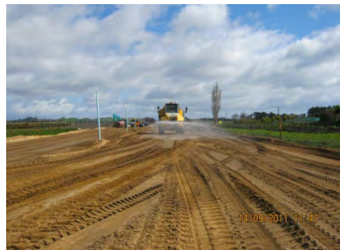
Figure 129: Water truck dampening down the works area
