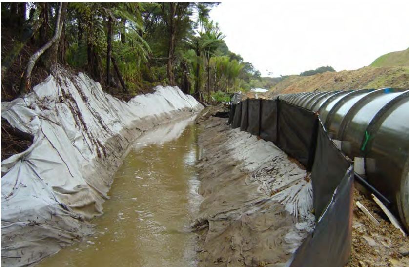
Figure 112: Temporary stream diversion to allow for the installation of a new culvert
