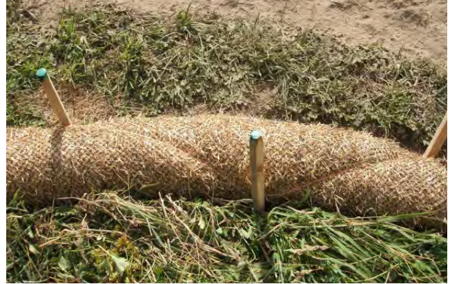
Figure 94: Straw sock secured in place using stakes and bale twine; note the stakes are placed every 600 mm
