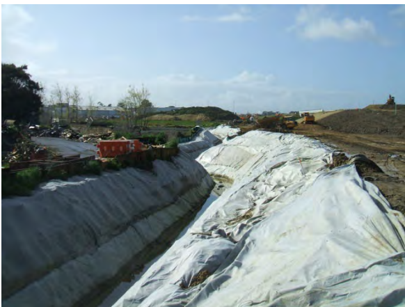
Figure 118: Examples of temporary stream diversion installed to allow permanent culverts to be installed off-line
