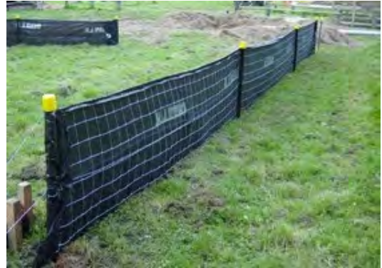
Figure 87: Super silt fence
