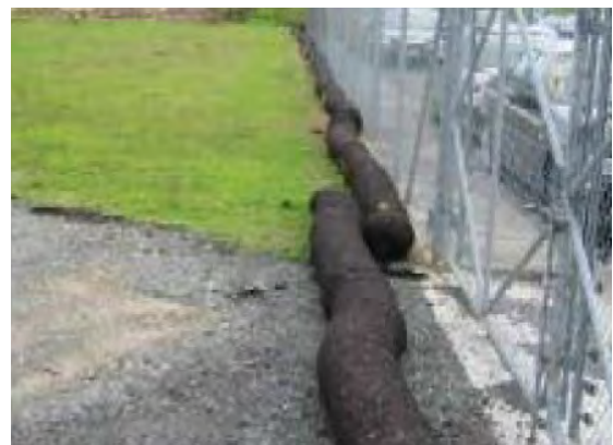
Figure 92: Silt sock with 1 m overlapping joint
