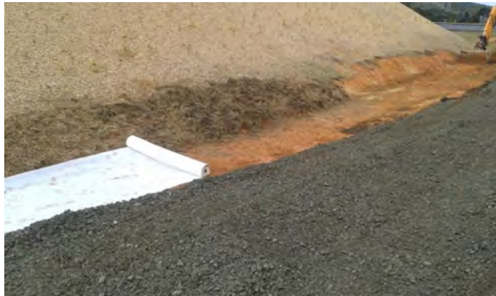
Figure 42: Stabilisation via a combination of chip mulch, geotextile and aggregate
