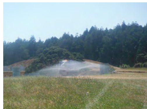
Figure 130: Regular wetting of the haul road
