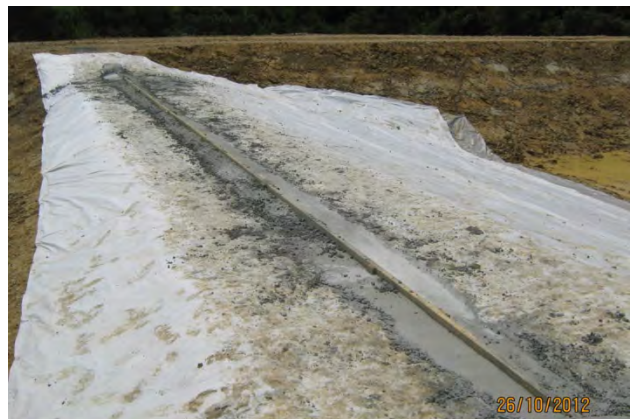
Figure 69: Example of a level spreader
