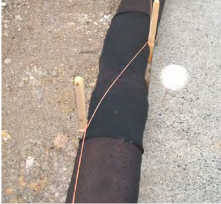
Figure 93: Silt sock joined using a sleeve and pegged and secured using baling twine with 1 m overlapping joint
