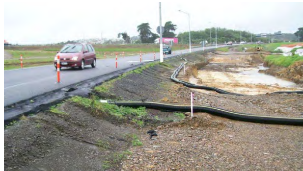
Figure 30: Flume conveying clean water over the works area
