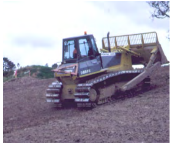
Figure 39: Surface roughening with bulldozer
