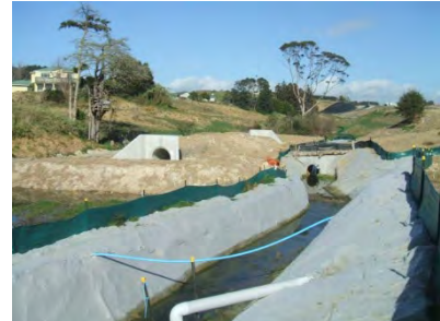
Figure 113: Stabilised clean water diversion and temporary culvert to divert streamflows while a new culvert is being constructed
