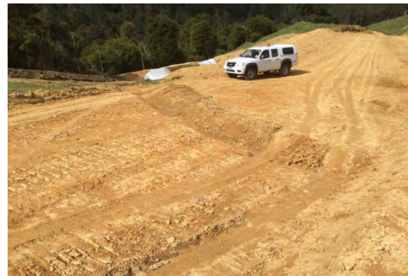
Figure 23: Contour drain installed across access track
