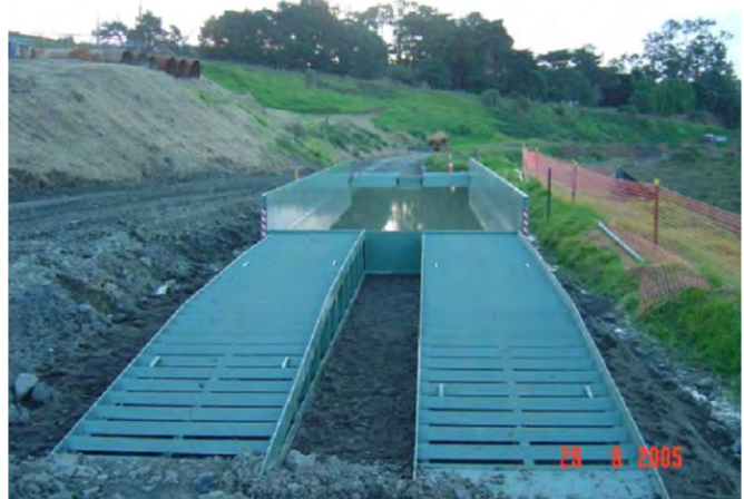
Figure 38: Example of a shaker ramp
