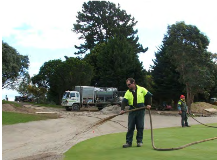
Figure 48: Specialist application of hydroseed
