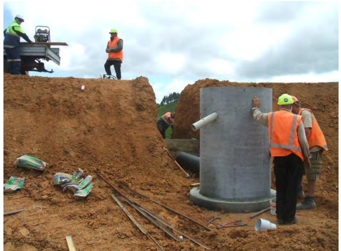
Figure 75: Installation of the outlet pipe and the anti-seep collars
