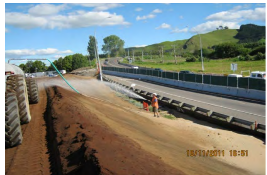
Figure 128: Dust suppression using soil binders/polymers
