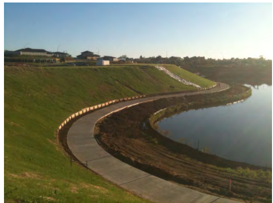
Figure 43: Grass stabilised earthworks site. Batter and building platforms
