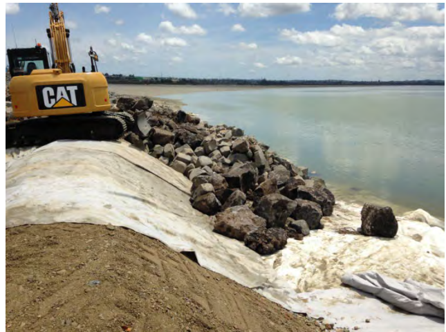
Figure 134: Use of geotextiles and coastal protection rock
