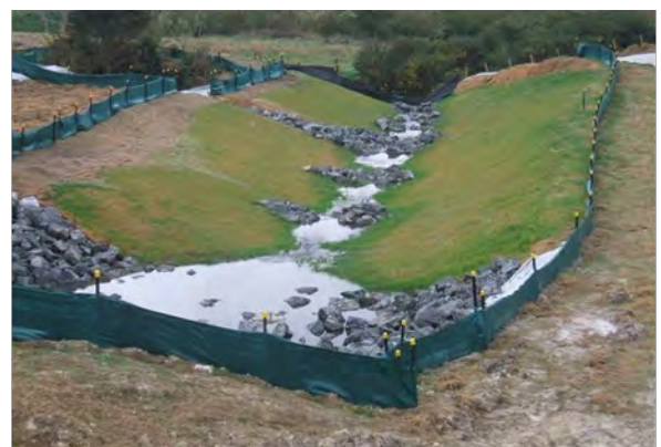
Figure 26: Check dams installed in series to act as a permanent water velocity control measure
