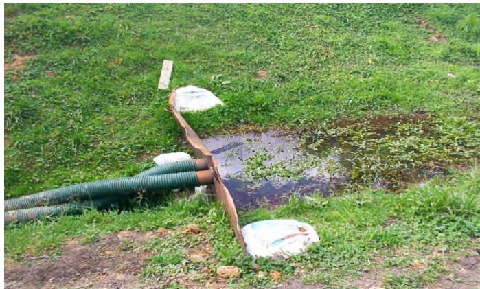
Figure 116: Water being diverted past a construction works area
