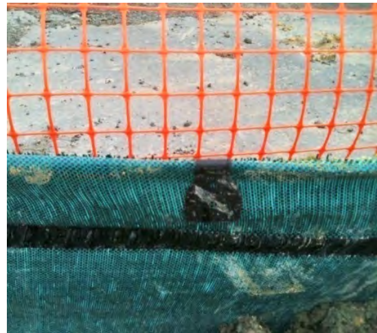
Figure 86: Use of silt fence clips
