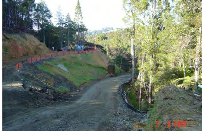
Figure 11: Northern Motorway construction site - minimising disturbance
