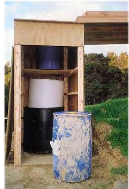
Figure 100: Rainfall activated flocculant treatment device
