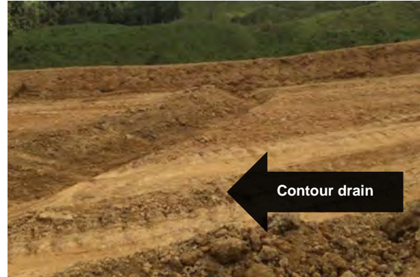
Figure 22: Contour drain
