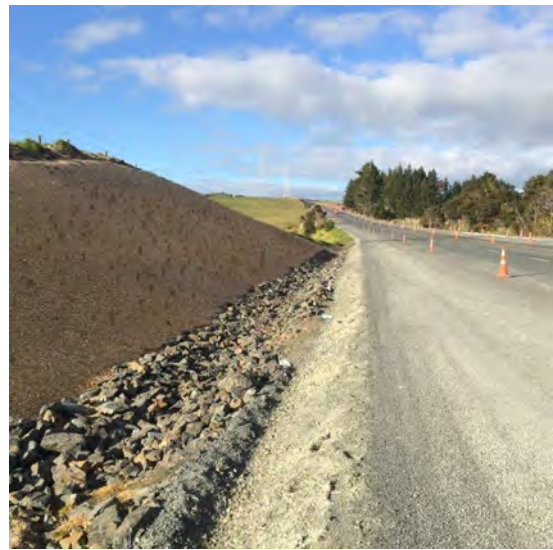
Figure 57: Woodchip to stabilise the finished batter slope
