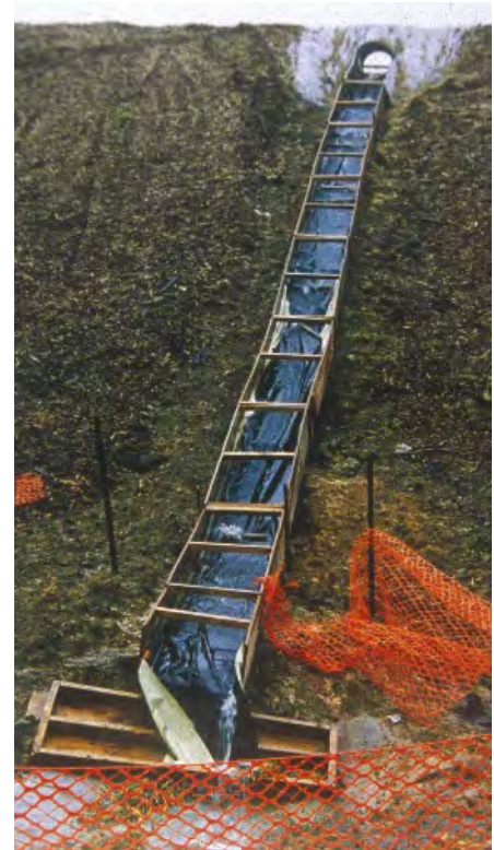
Figure 32: Wooden flume lined with impervious material
