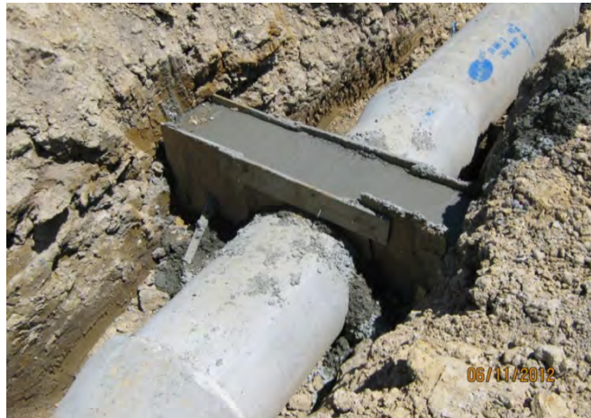
Figure 71: Example of an anti-seep collar
