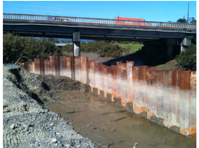
Figure 132: Sheet pile coffer dam
