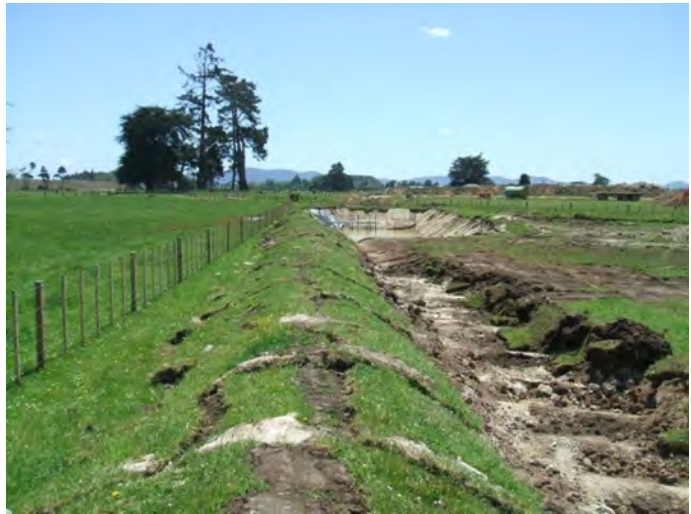
Figure 16: Turfing scraped from within the site to stabilise the perimeter bund. The perimeter bund provides both clean and dirty water control
