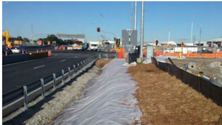
Figure 109: Progressive stabilisation in limited space
