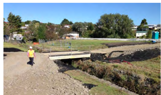
Figure 114: A temporary bridge in the process of being installed
