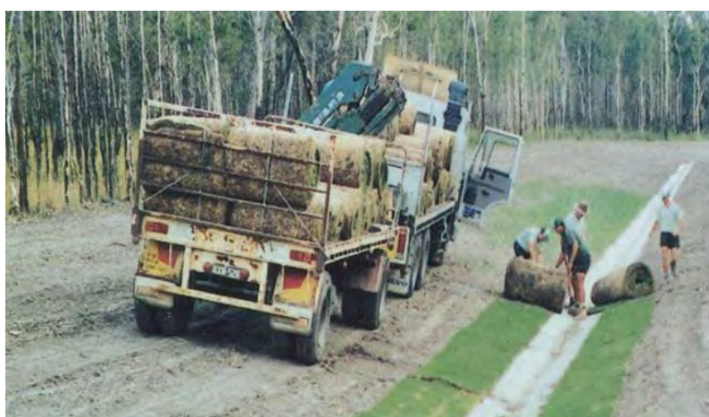
Figure 52: Turf being placed adjacent to a stabilised swale
