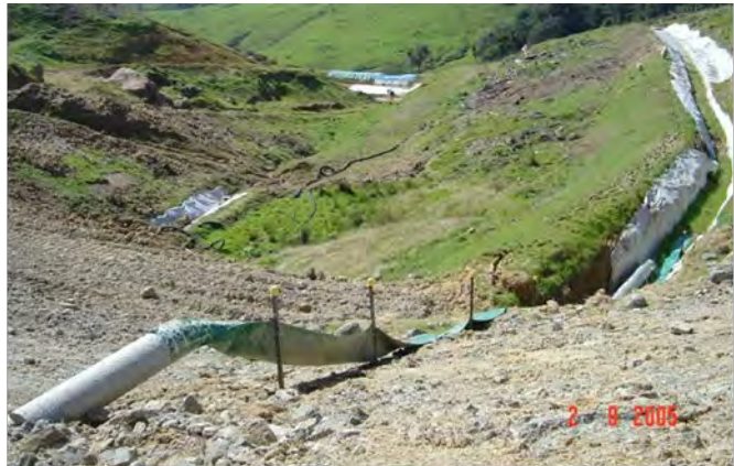
Figure 12: Flume installed to protect steep slope
