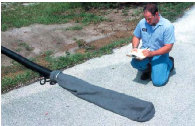
Figure 106: Dewatering bag and pipe sock
