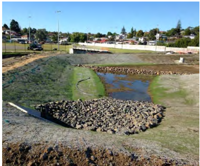
Figure 50: Recently applied hydroseed on a stormwater wetland
