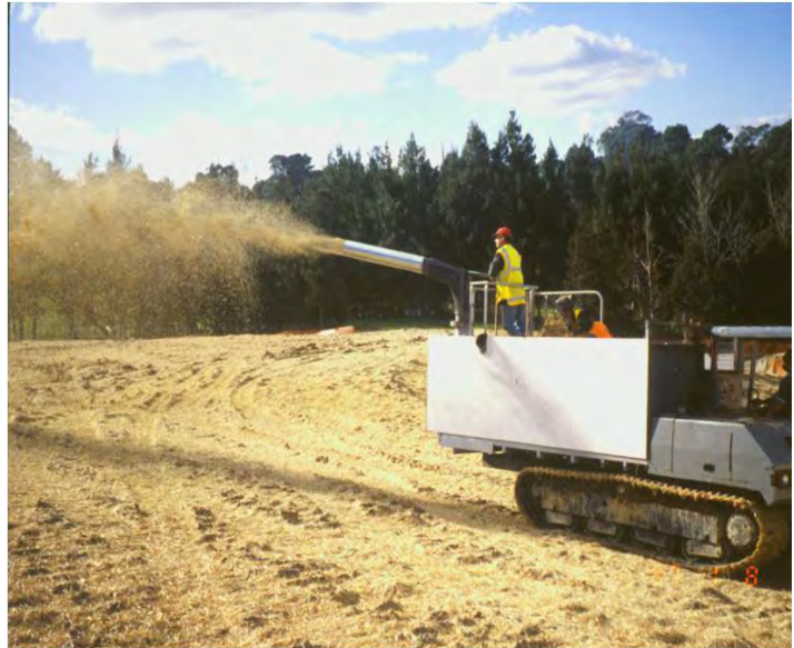
Figure 54: Specialist application of hay mulch
