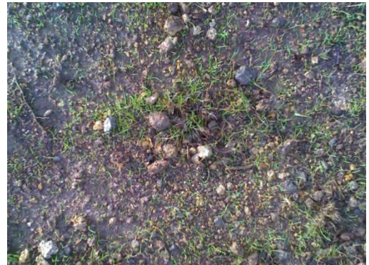
Figure 44: Initial grass strike - not stabilised
