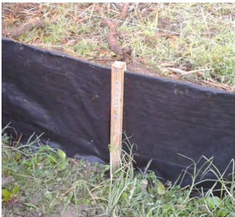
Figure 81: Silt fence joins. Left hand photo shows battens used to join the lengths. Right hand photo shows doubling over of fabric at end around the waratah
