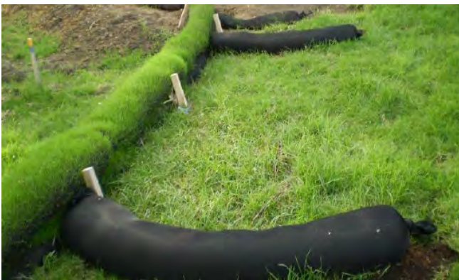
Figure 91: Compost silt socks with returns installed
