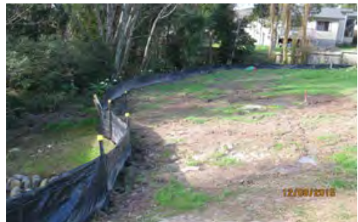
Figure 108: Silt fence
